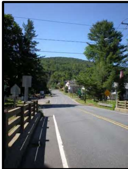
The bridge (with no sidewalks) on Jacksonville Road to the south of the Colrain Central School.
