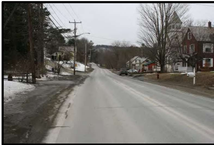
This view of Main Road near the Colrain Public Library shows the lack of sidewalk on this primary route in downtown.
